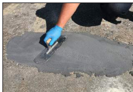
ARC EG-1 applied to concrete.
