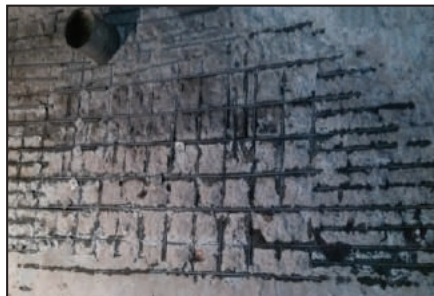
Chest wall after tile removed and blasted.
