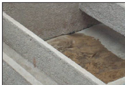
Drained sand filter vessel.
