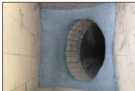
Installation of ARC BX5 .
