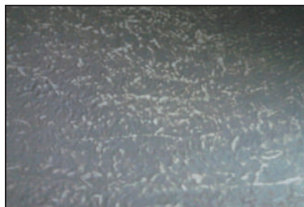
Corroded tank internal surface.
