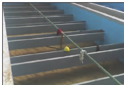
Installing ARC S1PW coating.
