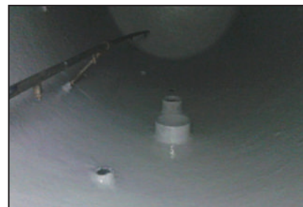
Coated tank internals.
