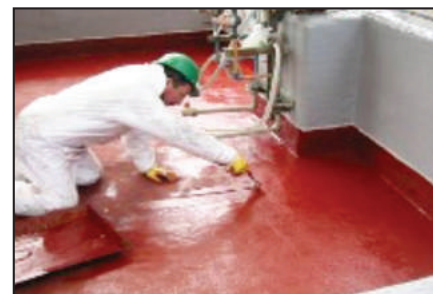
Applying ARC CS4 topcoat.
