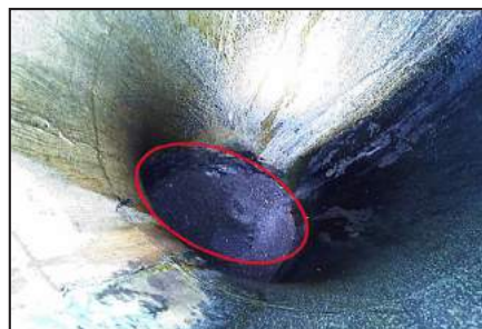
Dark scale formation on unlined section.
