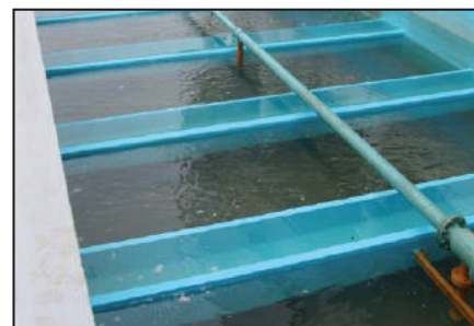
Sand filter in service.
