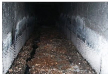
Discharge flume with damaged tile/rubber liners.
