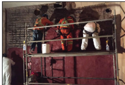
Installing ARC NVE coating.
