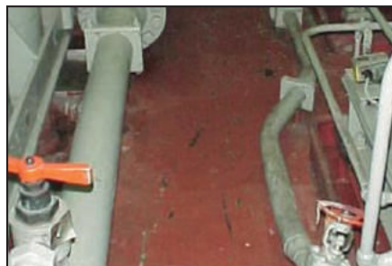
Previous coating one year after installed.
