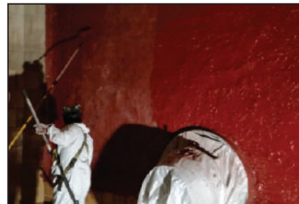
Applying ARC NVE sealer coat.
