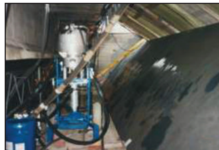
Pitting repaired using ARC 858 .
