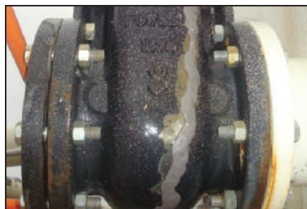
Valve leakage plugged with ARC 5ES.
