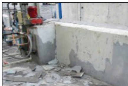
Failed coating after spills.
