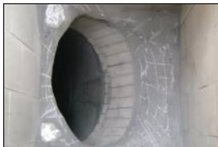
Damage to existing ceramic tiles caused by unscheduled shutdown and loss of production.
