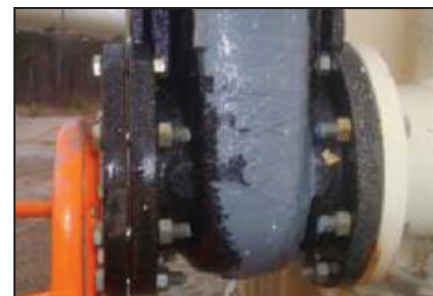
Repaired valve with ARC 5.
