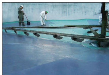
Alternating colors of ARC S2 .
